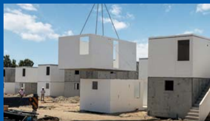
Peru, 2nd Modular Housing Plant, upcrete® read more on pages 18 – 19
