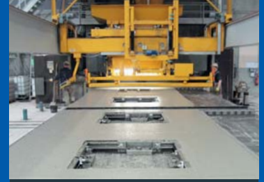
Denmark, Boligbeton Factory planning, general contractor
