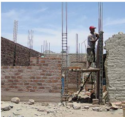
Example of conventional construction in Peru
