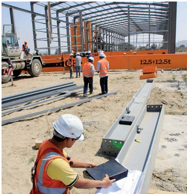
Even the foundations are prefabricated on-site.
