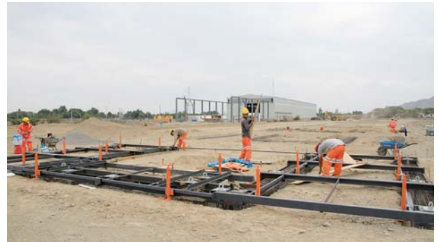
Even the foundations are prefabricated on-site.
