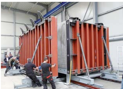
Opening the module formwork
